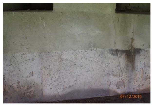
View of vertical cracking in the face of abutment 6 up to 0.026" wide under beam 4.
