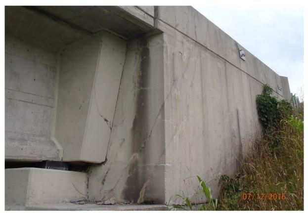
View of shear cracking with efflorescence and rust staining extending from the downstream wingwall (Wingwall A per plans) into the back-wall of the upstream face of abutment 1.
