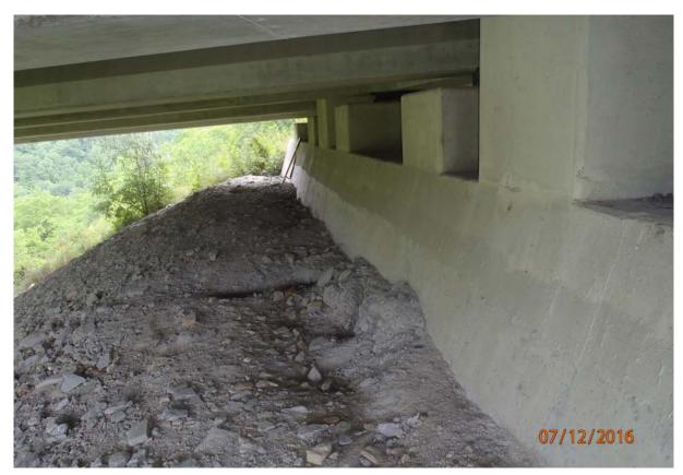
View along the face of abutment 1. Note the evidence of settlement and potential drag-down.
