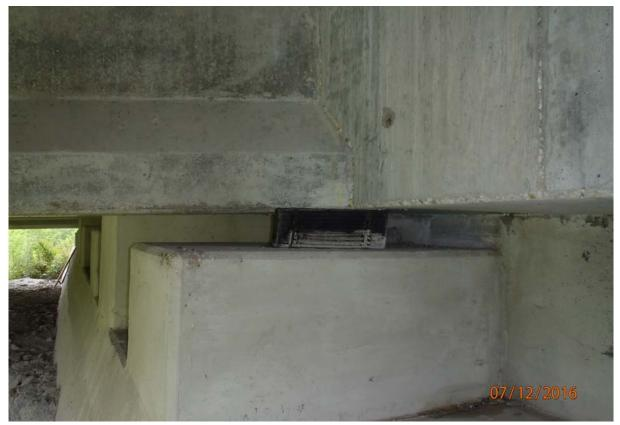
View of the bearing under beam 5 at abutment 1. Note the bearing pad has moved from its original position.
