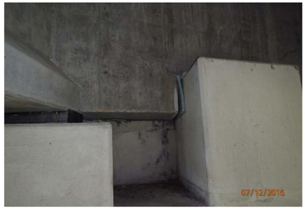
View of the horizontal gap between the diaphragm and shear block between beams 4 and 5 at abutment 1; indicating the superstructure has moved towards the upstream at this location.
