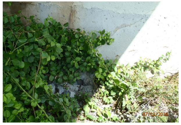
View of small void under the pile cap upstream of beam 1; no piles where exposed/detected.
