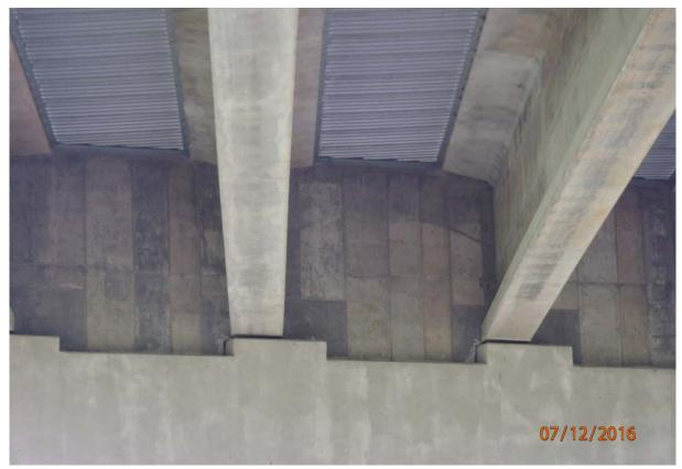
View of the south face of the diaphragm and superstructure of span 1 at pier 2. Note the gap between the diaphragm and beam seats indicating the superstructure has moved towards the downstream.
