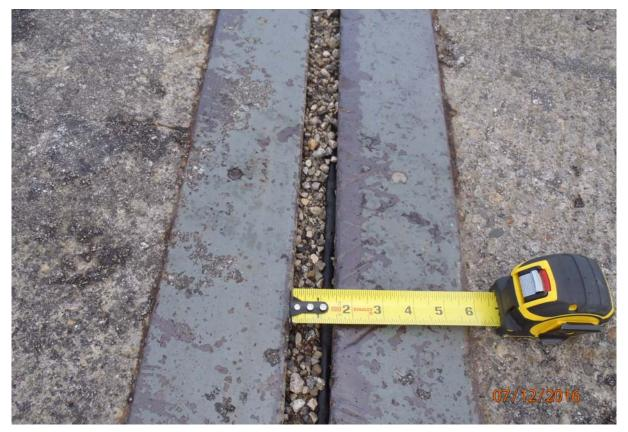
Close up view of the joint gap in the northbound lane at abutment 1.
