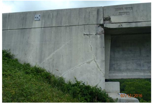
View of the downstream wingwall of abutment 6 (Wingwall C per plans). Note the spalling of the barrier wall, spalling of the wingwall, and shear cracking with efflorescence and rust staining up to 0.023" wide.
