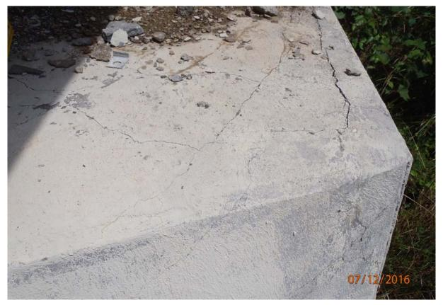
View of cracking present on the abutment seat upstream of beam 1. Note the cracking widths are up to 1/4" wide.
