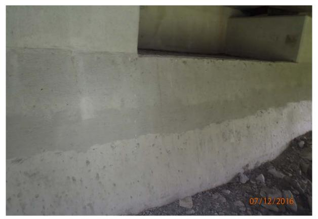
View of typical minor vertical cracking under the beam seats and spaced throughout between the beam seats of abutment 1.
