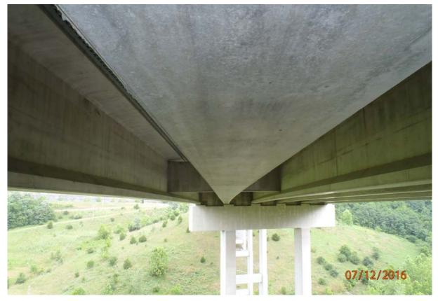
View sighted along the underside of beam 5 in span 1. Note it appears the beam is sweep towards the downstream.
