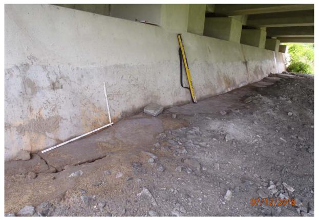
View along the face of abutment 6. Note at some point in the past heavy erosion was present exposing many of the piles at this abutment thus flow-able-fill was placed in the voided areas; the cracking and 22/75 settlement of the flow-able-fill finished surface indicates that settlement is continuing.
