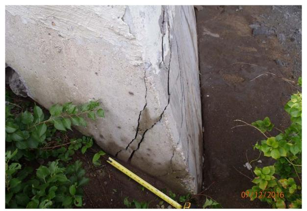
View of heavy cracking present at the downstream corning of the pile cap of abutment 6. Note the cracking is up to 1/2" wide.
