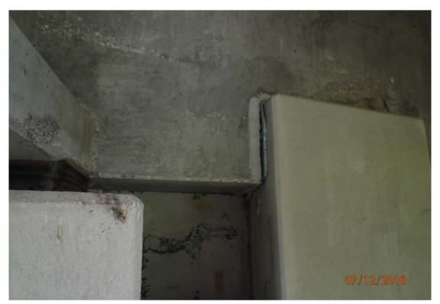
View of the shear key and diaphragm between beams 4 and 5 at abutment 6. Note the gap/movement of the superstructure towards the downstream.
