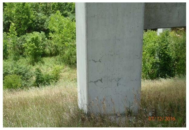
View of minor cracking on the north face of the upstream column of pier 5.
