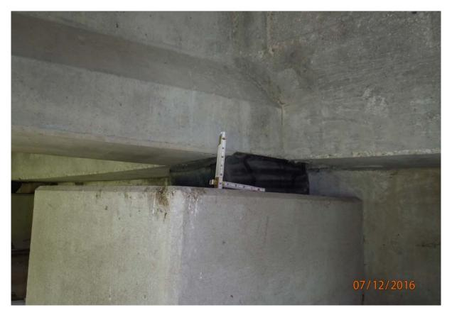
View of the bearing pad under beam 3 at abutment 6. Note the deformation and cracking.
