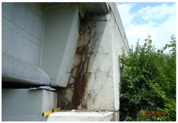
View of the back-wall upstream of beam 1. Note the heavy cracking up to 0.03" wide with efflorescence and rust staining. Note the green circles and PK nails - the below level reading was recorded at this location.
