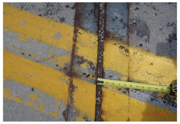
Close up view of the joint gap at the centerline of abutment 6.
