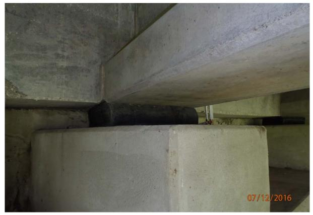
View of the bearing pad under beam 4 at abutment 6. Note the deformation and cracking.
