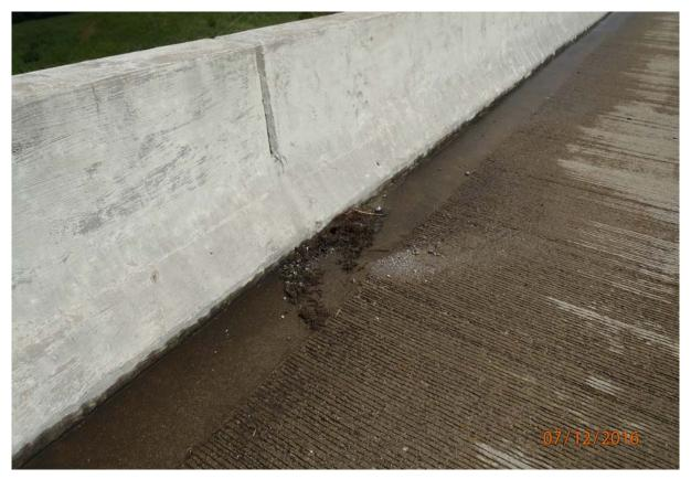
Some of the deck-drains are open, however a large number are 100% blocked with debris as shown above.
