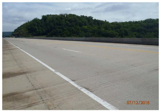
Typical view of the deck. Note minor there are minor to moderate transverse and longitudinal cracks throughout.
