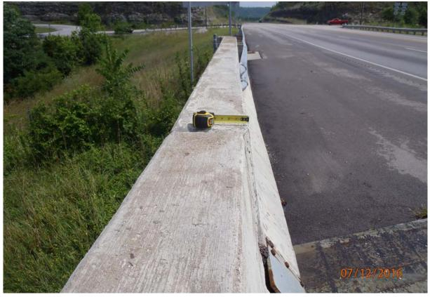
View of the horizontal offset between the downstream barrier wall at abutment 6. Note the entire superstructure appears to have moved towards the downstream at this location.
