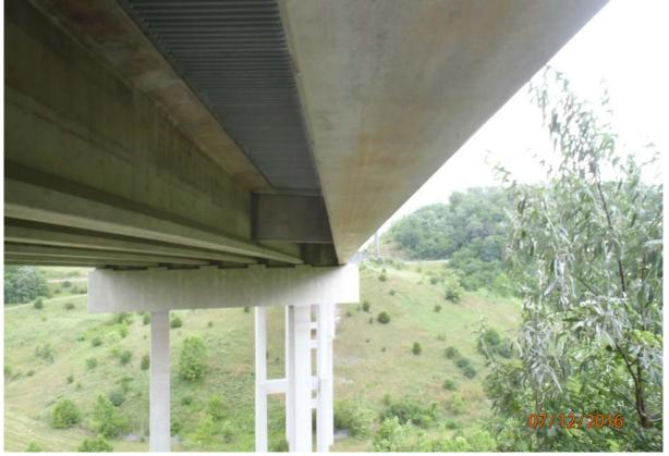
View sighted along the underside of beam 1 in span 1. Note it appears the beam is sweep towards the downstream.
