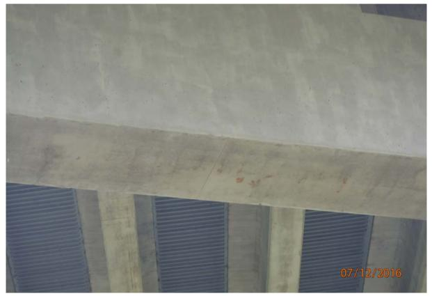
View of the underside of the pier cap of pier 5. Note the transverse rust staining most likely from inadequate cover over the stirrup/shear **47/75** reinforcing on cap underside.
