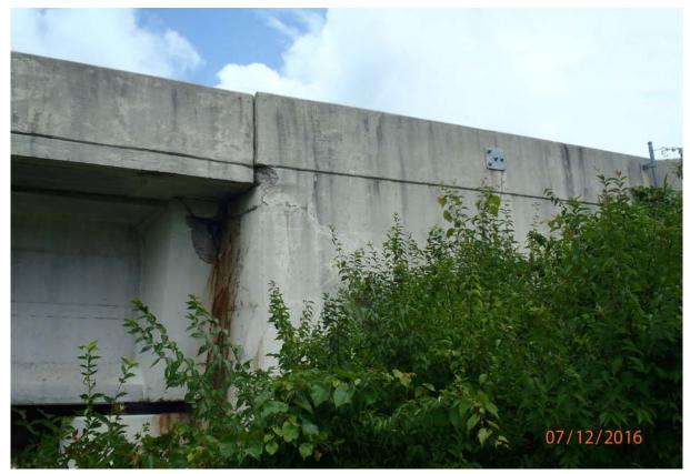
View of the upstream face of beam 1 at abutment 6. Note the heavy cracking and staining of/on the abutment back-wall, spalling of the diaphragm, and the cracking/spalling of the wingwall.
