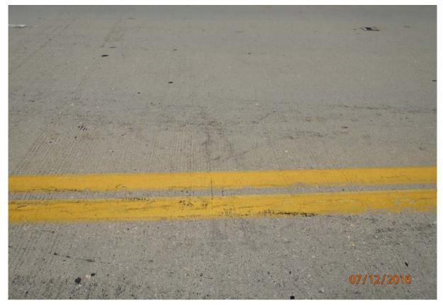
Close-up of transverse cracking noted in the bottom photo of page 10. Note this location is located at the beam ends over pier 2 of beamline 3.
