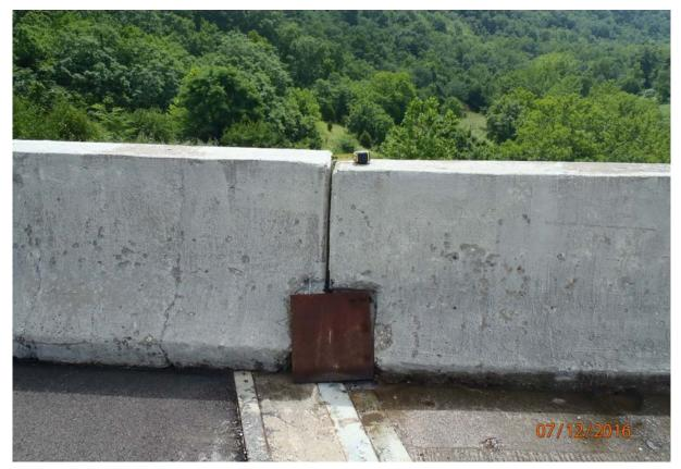
View of lateral offset between the upstream barrier wall at abutment 6. Note the barrier wall sliding plate has mostly torn off due to the horizontal and laterial movement.
