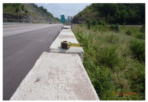
View of the horizontal offset between the upstream barrier wall at abutment 6. Note the entire superstructure appears to have moved towards the downstream at this location. **16/75**
