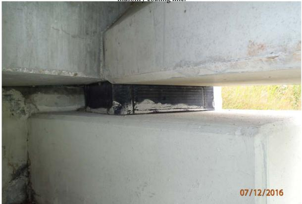
View of the bearing under beam 6 at abutment 1. Note the bearing pad has moved from its original position.
