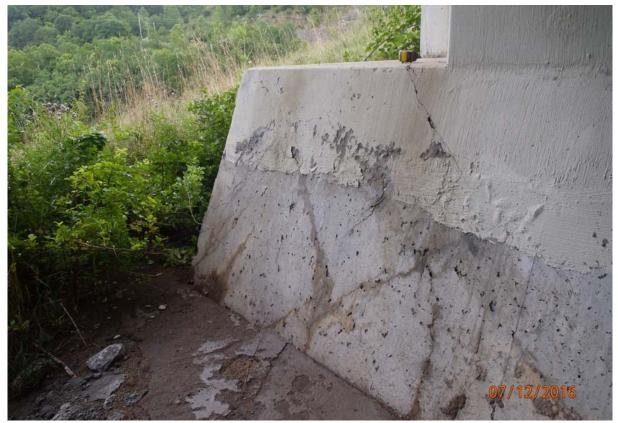
View of the face of the pile cap under and downstream of beam 6. Note the heavy cracking with rust staining; the cracks are up to 0.02" wide at this location.
