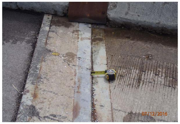
View looking down at the joint over abutment 6 near the upstream barrier wall. Note the joint is completely closed at this location.
