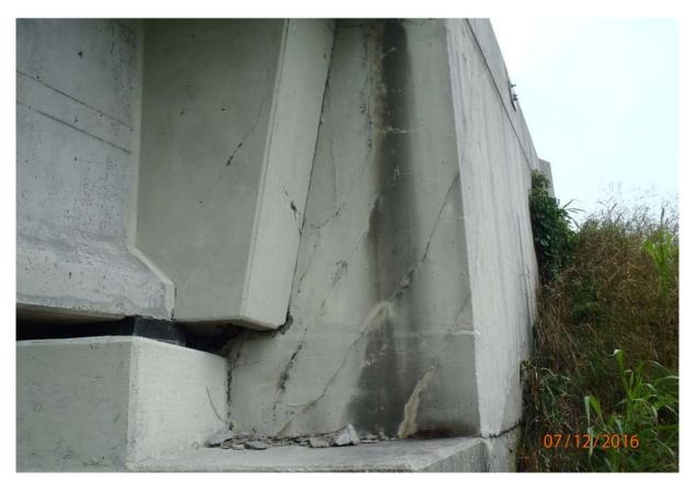
View of the back-wall downstream of beam 6. Note the cracking in the back.
