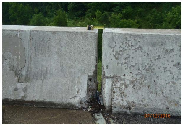
View of lateral offset between the upstream barrier wall at abutment 1. Note the barrier wall sliding plates have torn off due to the horizontal movement.
