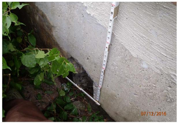
View of a spall and void under the downstream side of the pile cap of abutment 6. Note no piles are exposed but reinforcing steel is without any measureable section loss.
