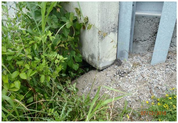
View of erosion under the approach roadway slab located at on upstream side near abutment 6.
