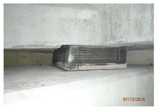
View of the bearing under beam 3 at abutment 1. Note the bearing pad has moved from its original position.
