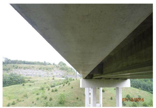
View sighted along the underside of beam 6 in span 1. Note it appears the beam is sweep towards the upstream.
