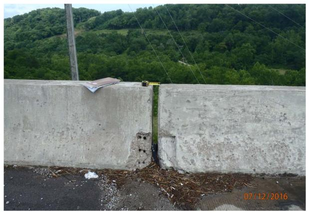
View of lateral offset between the downstream barrier wall at abutment 1. Note the barrier wall sliding plates have torn off due to the horizontal movement.
