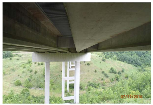
View sighted along the underside of beam 2 in span 1. Note it appears the beam is sweep towards the downstream.
