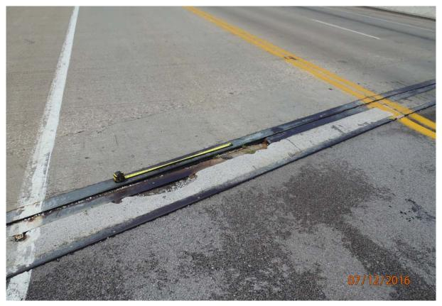
View of snowplow damage to joint at abutment 6, in the northbound lane.
