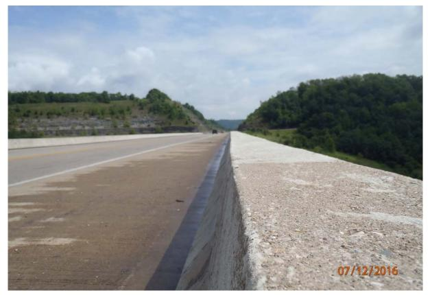
View sighted along the upstream barrier wall looking from abutment 1. Note the top of the wall appears to be wavy throughout, this is consistent with the driving surface; traffic appears to bounce while crossing the structure in both directions.
