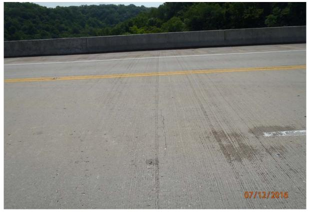
View of transverse cracking in the deck over at one line of the beam ends over pier 2.
