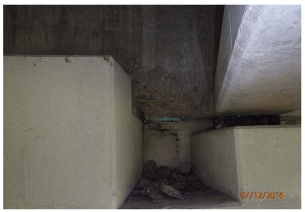
View of the diaphragm and shear block between beams 4 and 5 (beam 5 on right). Note the diaphragm is spalled with exposed reinforcing steel without section loss. In addition note the **63/75** superstructure is pressed tight against the abutment back-wall the entire length of the abutment.
