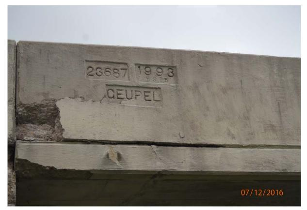
View of the date, design loading, plan number, and contractor stamp located on the upstream face of the downstream barrier wall at abutment 6.
