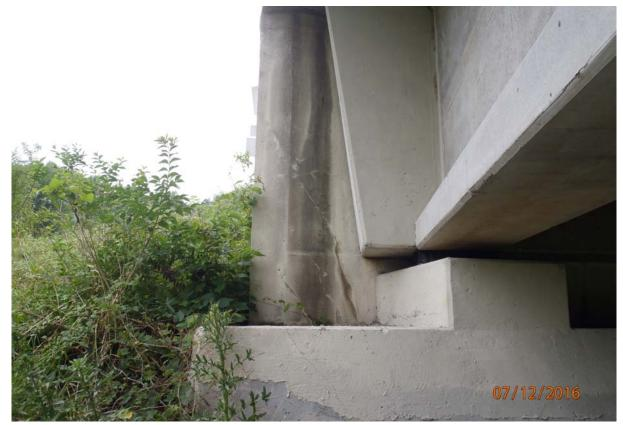
View of the back-wall upstream of beam 1. Note the cracking in the back.
