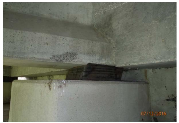
View of the bearing pad under beam 5 at abutment 6. Note the deformation and cracking.
