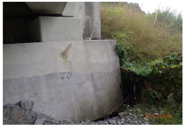
View of erosion and voided area/undermining of the downstream side of the pile cap of abutment 1 at/near beam 1. No piles are exposed or could be detected.
