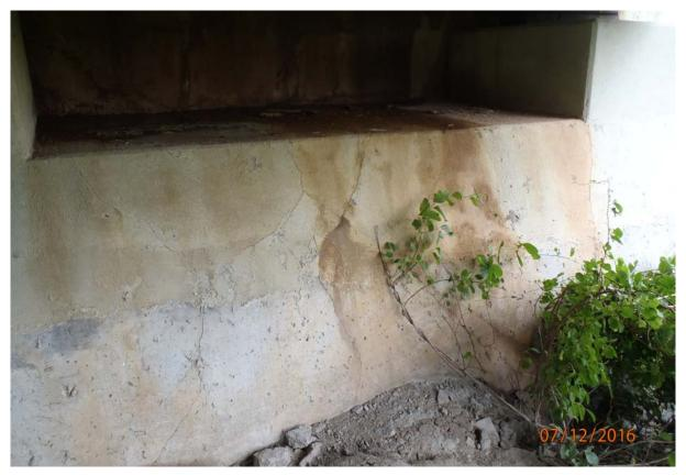
View of cracking in the face of abutment 6 between beams 1 and 2.
