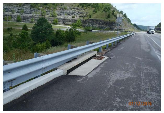
View of the downstream approach roadway drain at the end of the north approach slab (typical of the upstream at this location).
