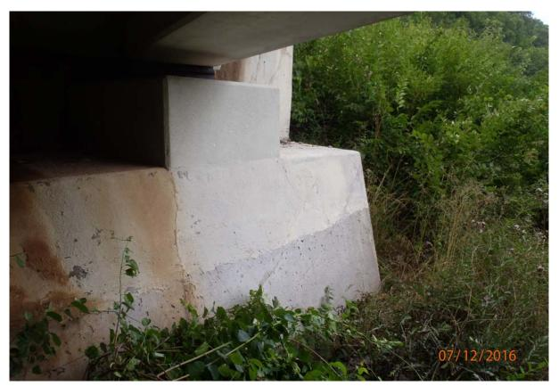
View of cracking under beam 1, upstream of beam 1, and downstream of beam 1 in the face of abutment 6.
