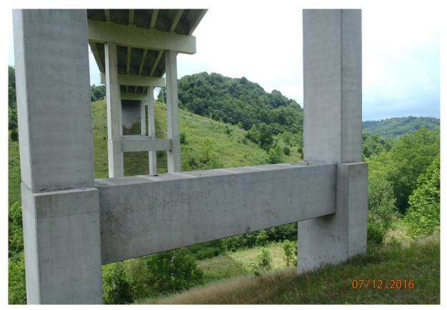
View of the strut of pier 5. Note the evidence of diaphragm spalling located on the top of the strut.
