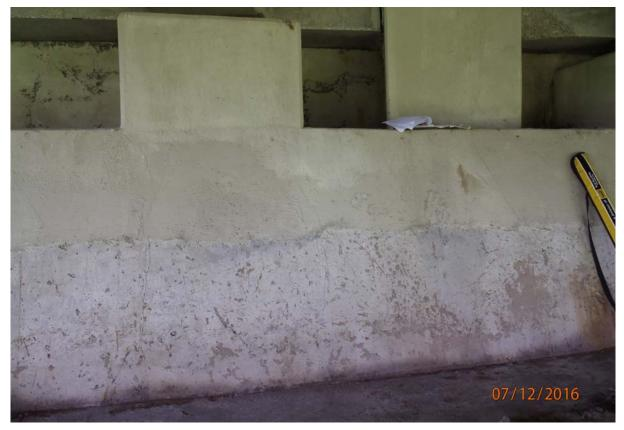
View of vertical cracking in the face of abutment 6 under and between beams 4 and 5; up to 0.05" wide under beam 5 and up to 0.03" wide between beams 4 and 5.
