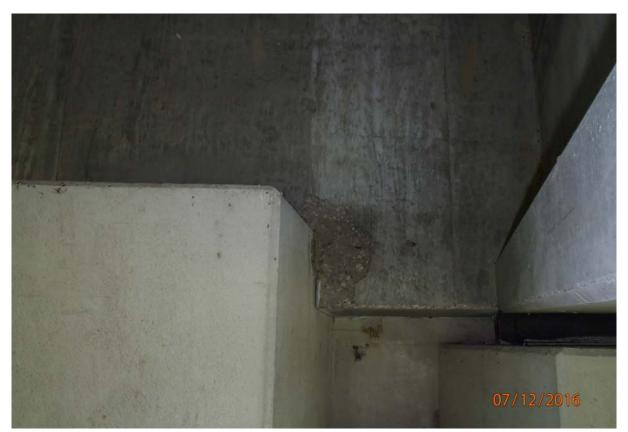
View of the diaphragm and shear block between beams 2 and 3 (beam 3 on right). Note the diaphragm is spalled.
