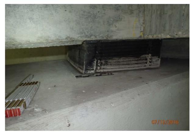
View of the bearing under beam 5 at abutment 1. Note the bearing pad has moved from its original position.
