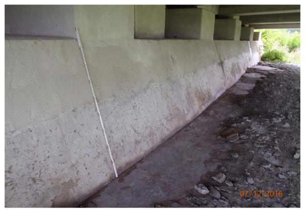
View of 2'-5" of vertical difference between the constructed height of the fill along abutment 6. Note photos dated back to 1997 indicate that the fill was approximately to/near the masonry coating line.
