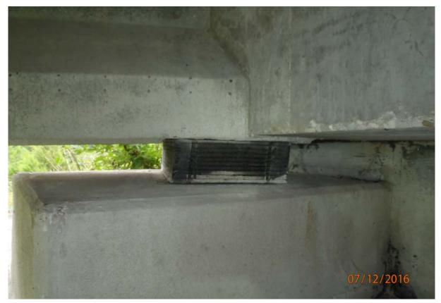
View of the bearing under beam 1 at abutment 1. Note the bearing pad has moved from its original position.
