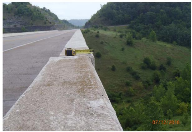
View of the horizontal offset between the upstream barrier wall at abutment 1. Note the entire superstructure appears to have moved towards the upstream at this location.
