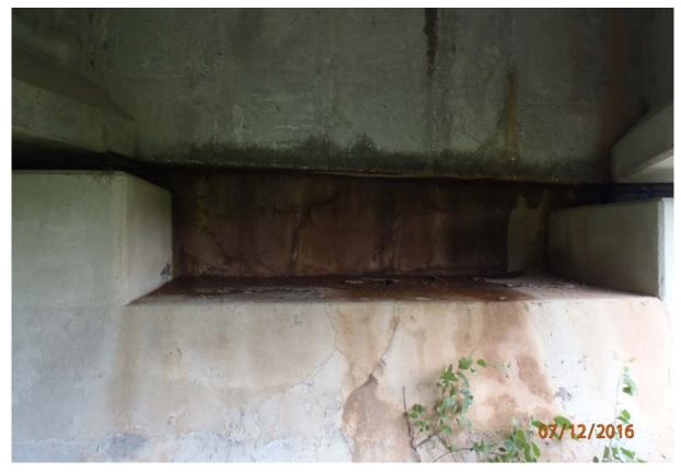
View of cracking and heavy staining in the back-wall of abutment 6 between beams 1 and 2.
