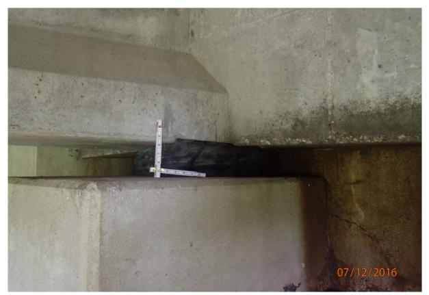
View of the bearing pad under beam 2 at abutment 6. Note the deformation and cracking.
