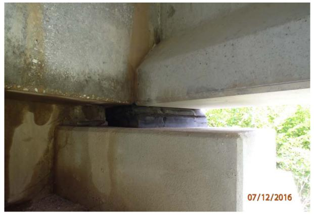
View of the bearing pad under beam 1 at abutment 6. Note the deformation and cracking.
