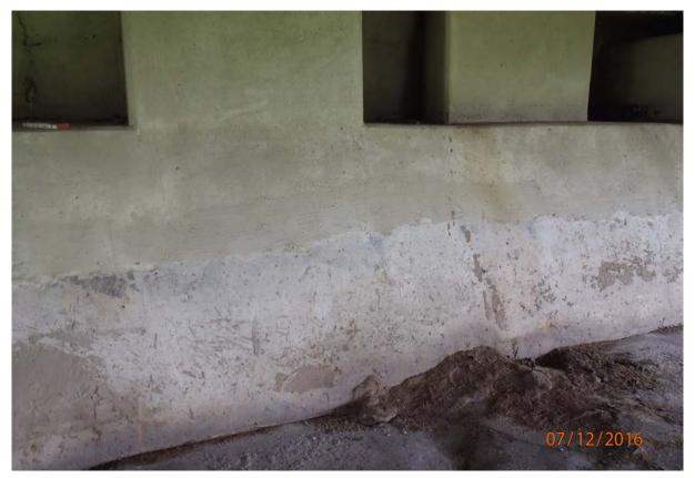
View of cracking in the face of abutment 6 under beam 3.
