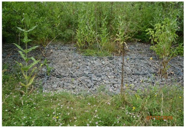
Close-up of gabion baskets at the base of the fill (around pier 4) of the north fill/embankment.
