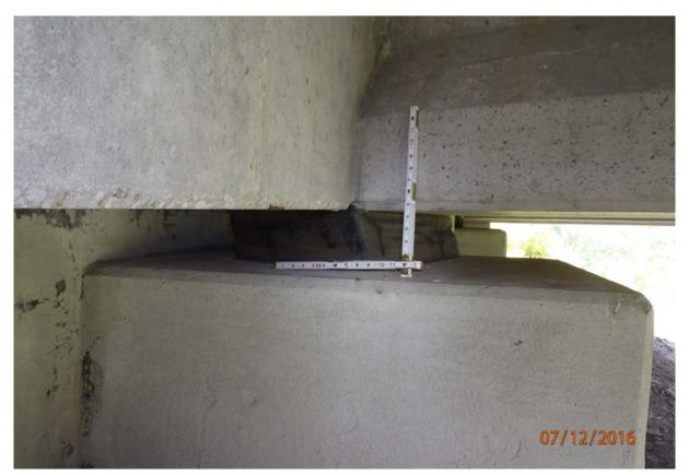
View of the bearing pad under beam 5 at abutment 6. Note the deformation and cracking.
