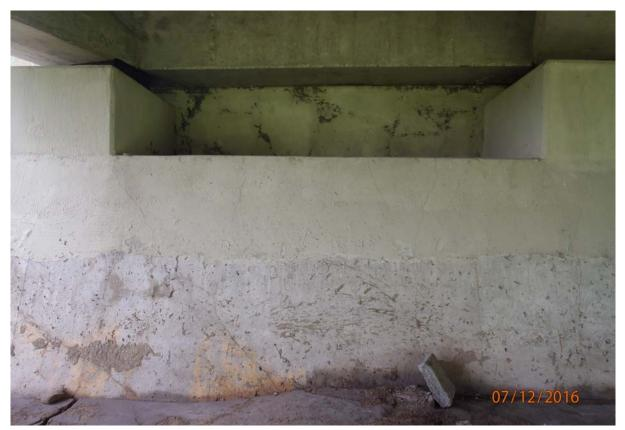
View of vertical and diagonal cracking in the back-wall and abutment face between beams 5 and 6 at abutment 6. Note the cracks in the abutment face are up to 0.023" wide, and some with rust staining.
