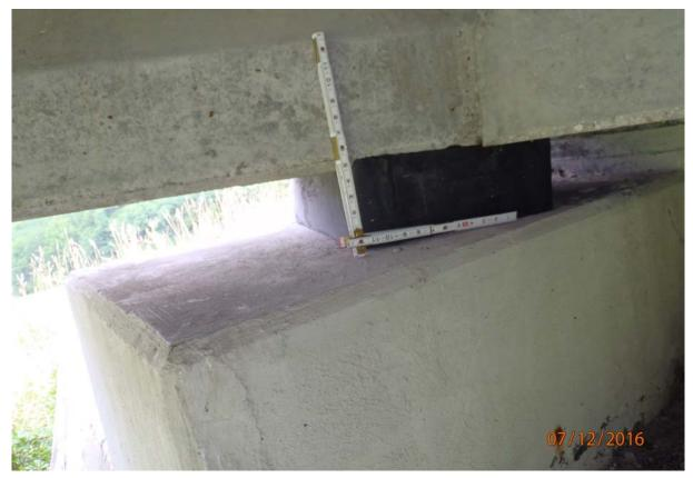
View of the bearing pad under beam 6 at abutment 6. Note the deformation and cracking.
