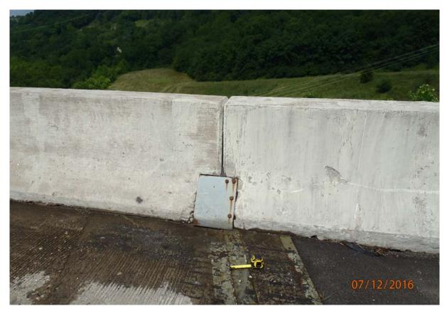
View of lateral offset between the downstream barrier wall at abutment 6. Note the deck joint is completely closed at this location.
