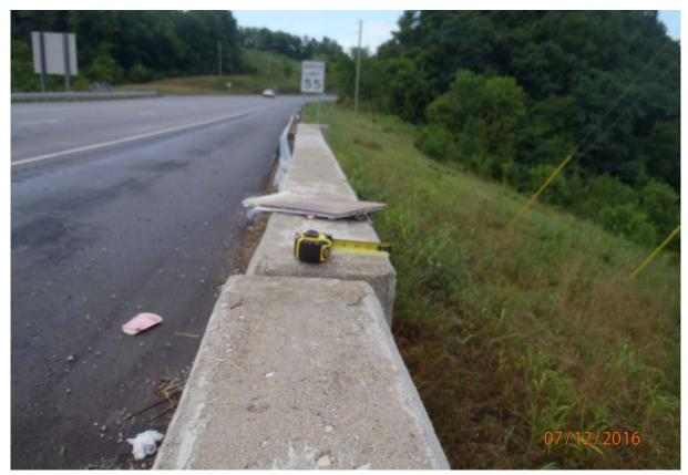
View of the horizontal offset between the downstream barrier wall at abutment 1. Note the entire superstructure appears to have moved towards the upstream.
