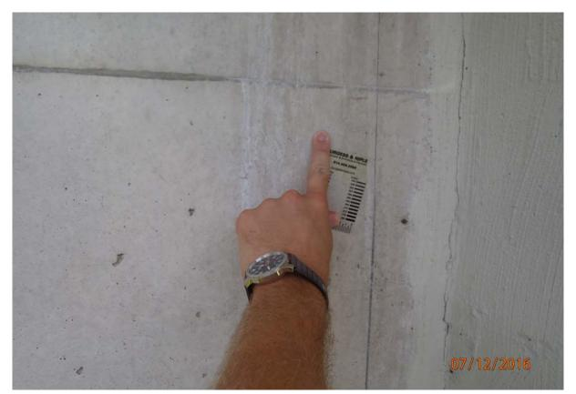
View of very minor longitudinal/diagonal cracks in the exterior face of beam 1 (3 cracks in total) extending from the diaphragm into span 5 approximately 15" from the face of the diaphragm; the cracks are up to 0.002" wide.
