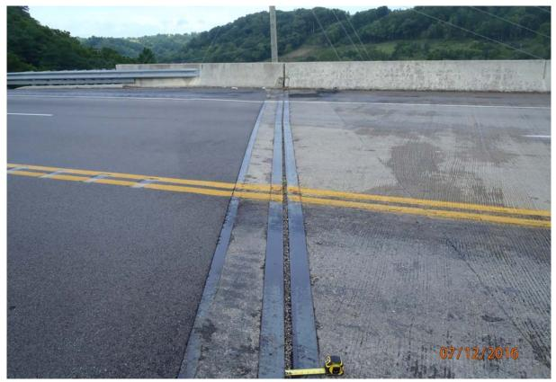
View looking down and along the deck joint of abutment 1. Note the joint is full of debris and compressed/closed past the anticipated/tolerable limits.
