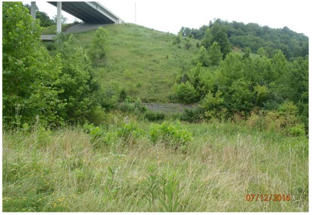
View of the fill/embankment on the downstream side of abutment 6. Note the gabion baskets at the base of the fill.
