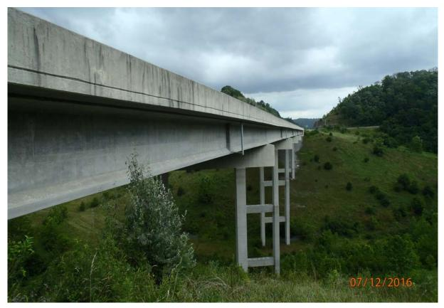
View along the upstream face of beam 6 looking from abutment 1. Note the waviness of the superstructure.
