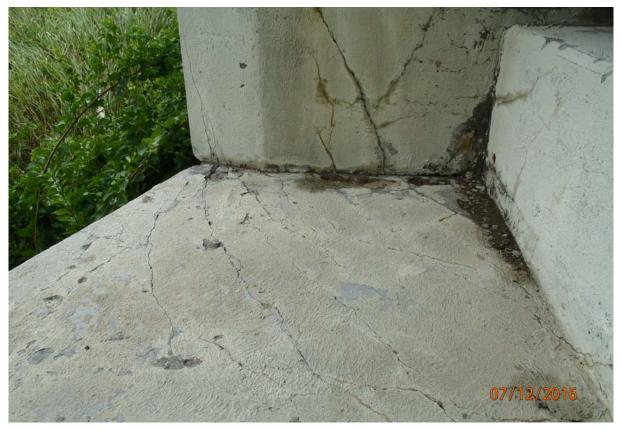
View of cracking present on the abutment seat downstream of beam 6. Note the cracking widths are up to 0.06" wide.
