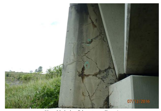
View of the back-wall downstream of beam 6. Note the heavy cracking up to 0.02" wide with efflorescence and rust staining. Note the green circles and PK nails - the below level reading was recorded at this location.
