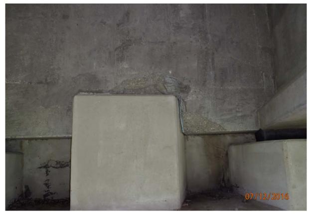
View of the shear key and diaphragm between beams 4 and 5 at abutment 6. Note the spalling of the back-wall.
