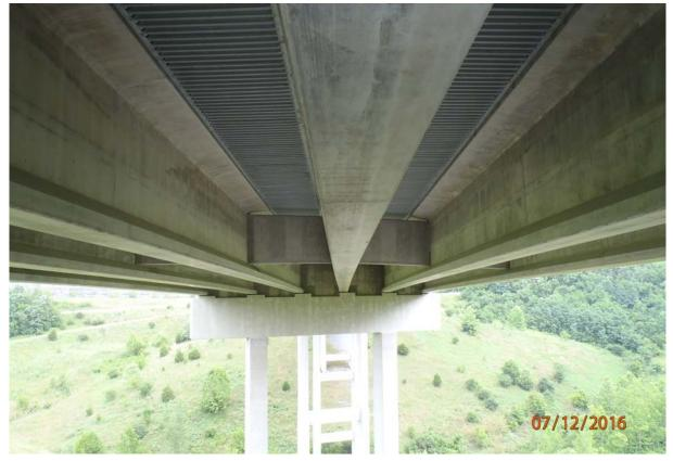
View sighted along the underside of beam 3 in span 1. Note it appears the beam is sweep towards the downstream.
