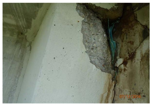
View of diaphragm and back wall spalling located upstream of beam 1. Note the diaphragm spall is approximately 20" tall with no exposed reinforcing steel.
