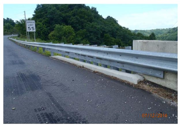
View of the downstream approach slab curb constructed in the recent asphalt roadway project (downstream similar).
