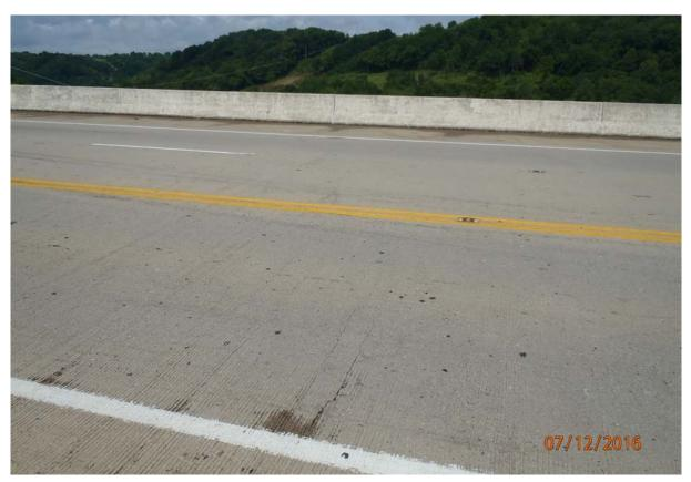
If you look closely, you can see the deck transverse cracking present at all of the interior beam ends over pier 2; note the cracking is aligned with the bridge skew.
