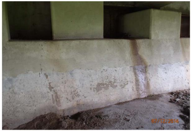
View of cracking in the face of abutment between beams 2 and 3.
