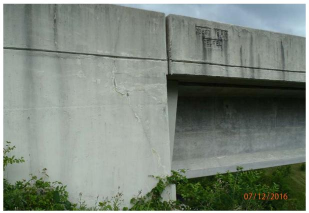
View the upstream wingwall of abutment 1 (Wingwall B per plans). Note the shear cracking with effloresce staining.
