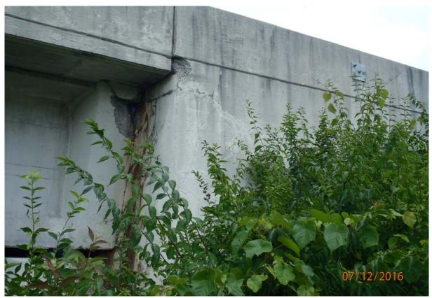
View of the upstream wingwall of abutment 6 (Wingwall D per plans). Note the spalling of the wingwall/back-wall, cracking of the back-wall, and shear cracking with efflorescence up to 0.023" wide.
