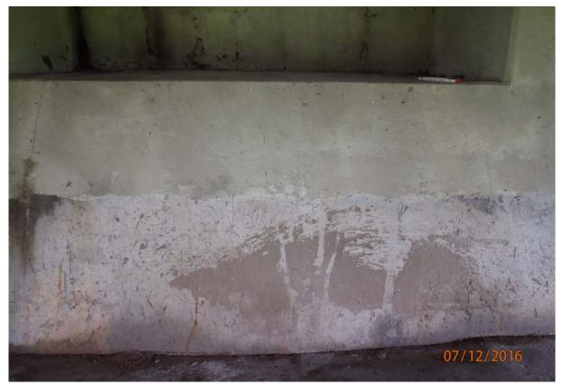
View of cracking in the face of abutment 6 between beams 3 and 4.
