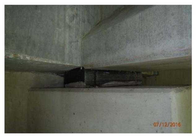
View of the bearing under beam 4 at abutment 1. Note the bearing pad has moved from its original position.
