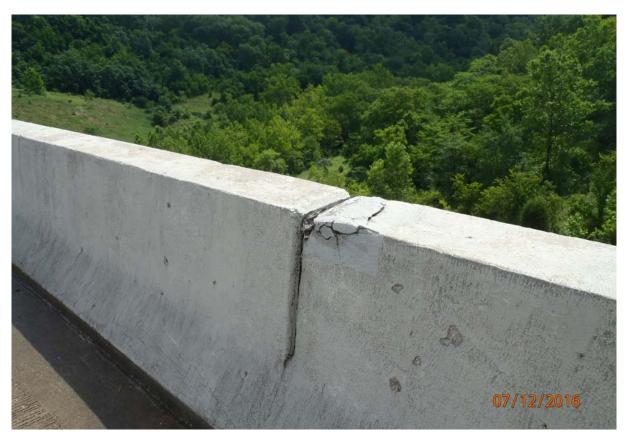
View of minor spall on the top of the upstream barrier wall located at the first drain from abutment 1 in span 1.
