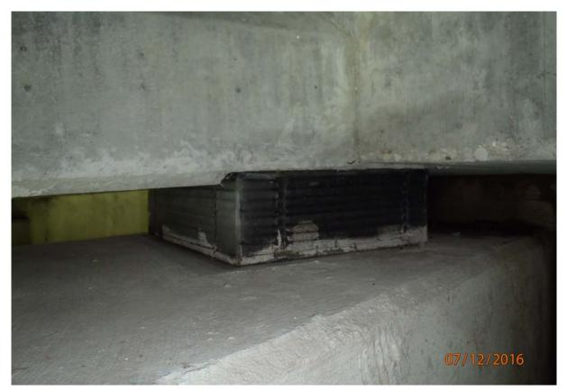
View of the bearing under beam 2 at abutment 1. Note the bearing pad has moved from its original position.
