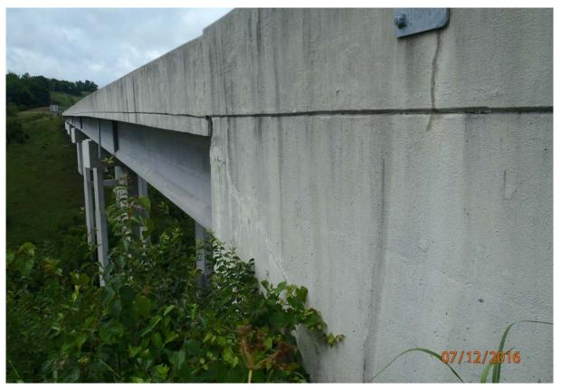
View along the upstream face of the upstream beam (beam 1) looking from abutment 6. Note the shear cracking in the wingwall (Wingwall D per plans). The shear cracks are up to **19/75** 0.023" wide with efflorscence staining.
