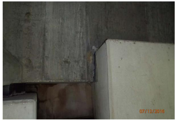
View of the horizontal gap between the diaphragm and shear block between beams 2 and 3 at abutment 1; indicating the superstructure has moved towards the downstream at this location.
