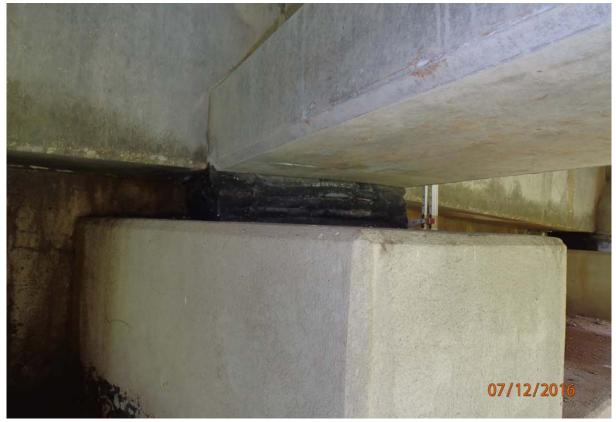
View of the bearing pad under beam 2 at abutment 6. Note the deformation and cracking.
