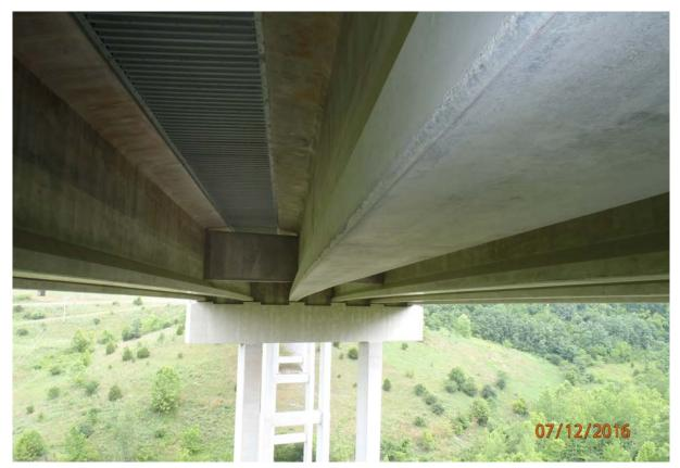
View sighted along the underside of beam 4 in span 1. Note it appears the beam is sweep towards the downstream.
