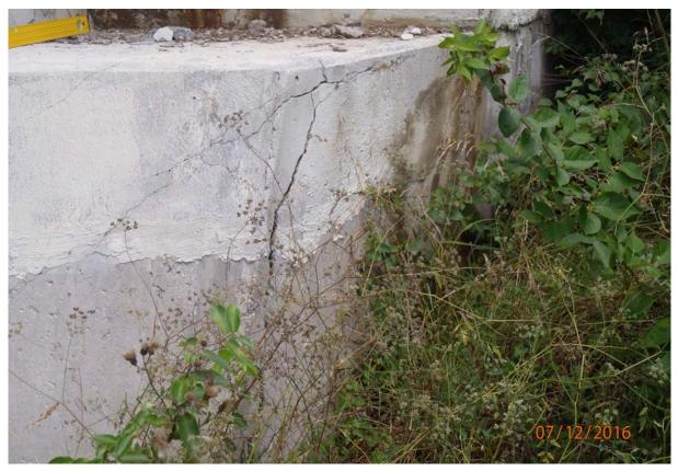
View of cracking present at the upstream corning of the pile cap of abutment 6. Note the cracking is up to 2" wide near the base of the pile cap with exposed reinforcing steel without section loss.
